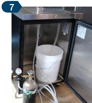
7 If using a gas tank , move it to the side. Place the drip tray drainage hose in a bucket with a minimum capacity of 5 gal.
